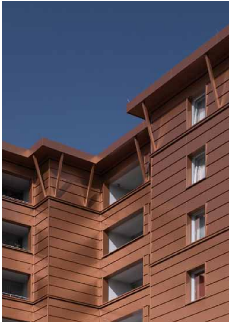
View of the »Italian« quarter: Upper roof edge made of ALUCOBOND® with a fascia forming the transition to the facade and support
